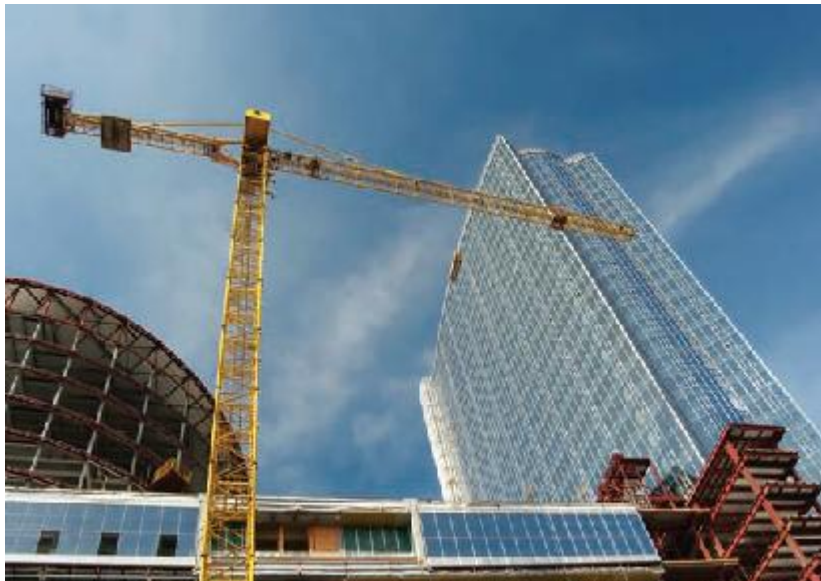
FIGURE 1-5 Construction crane on a building site (Shutterstock)
